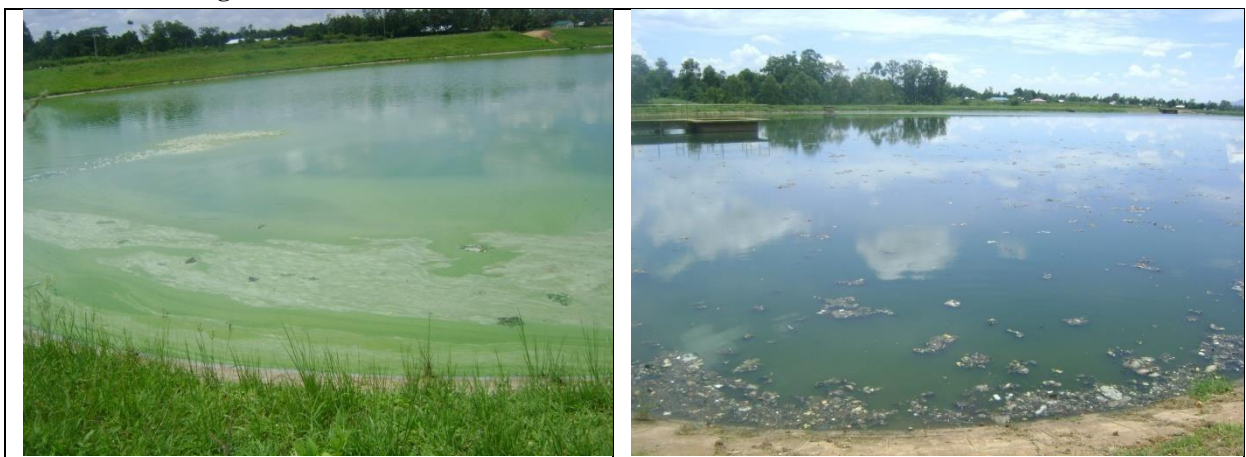
Sewerage ponds in Busia
