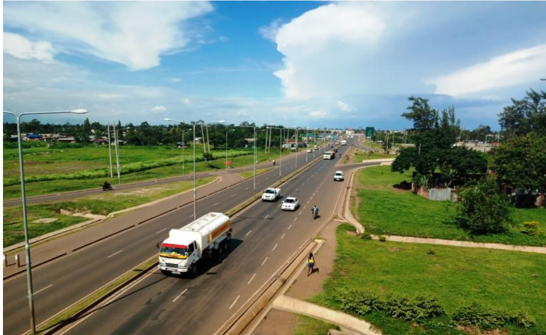
Plate 1: Intersection of Nyamasaria-Kondele Bypass with Kisumu-Kericho Road
