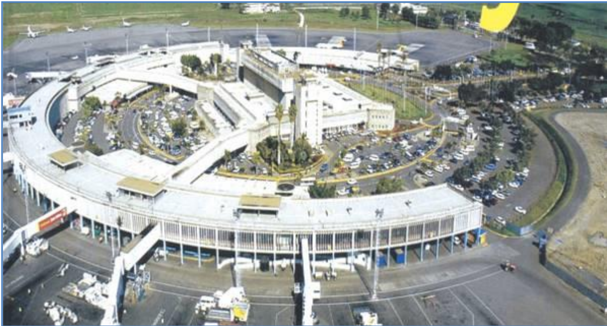
Plate 4: Jomo Kenyatta International Airport
