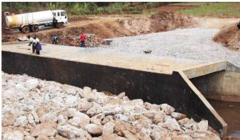
Figure 3: Rehabilitation of Mukuyu-Githambo-Kiruri Road
