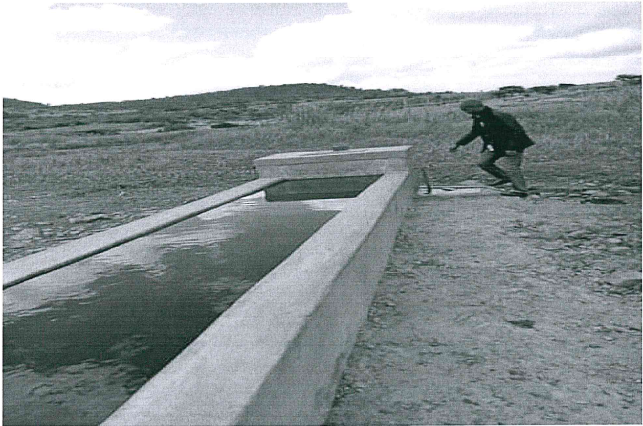
Rehabilitation of Gatami water intake in Muhotetu
