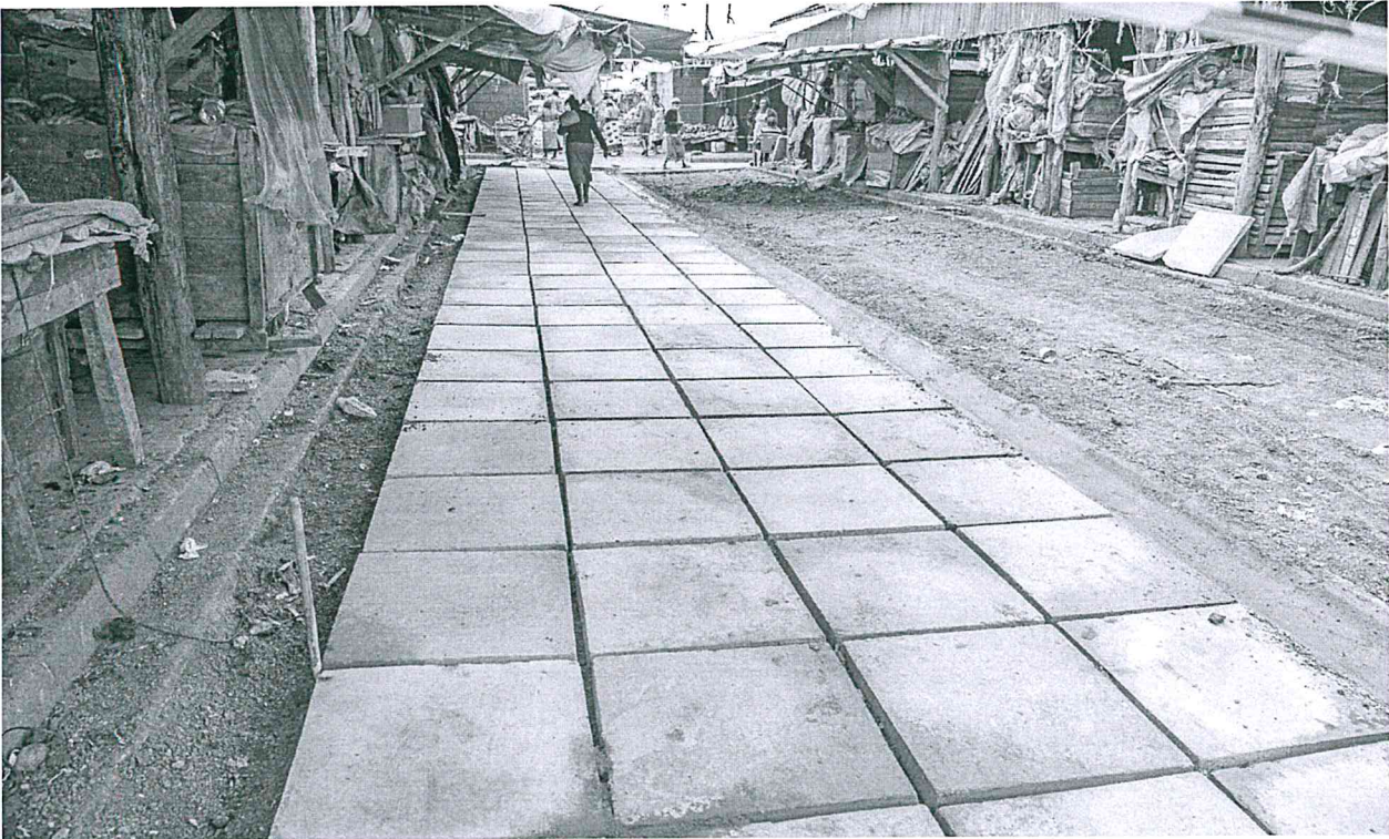
Marikiti market rehabilitation- Nanyuki ward
