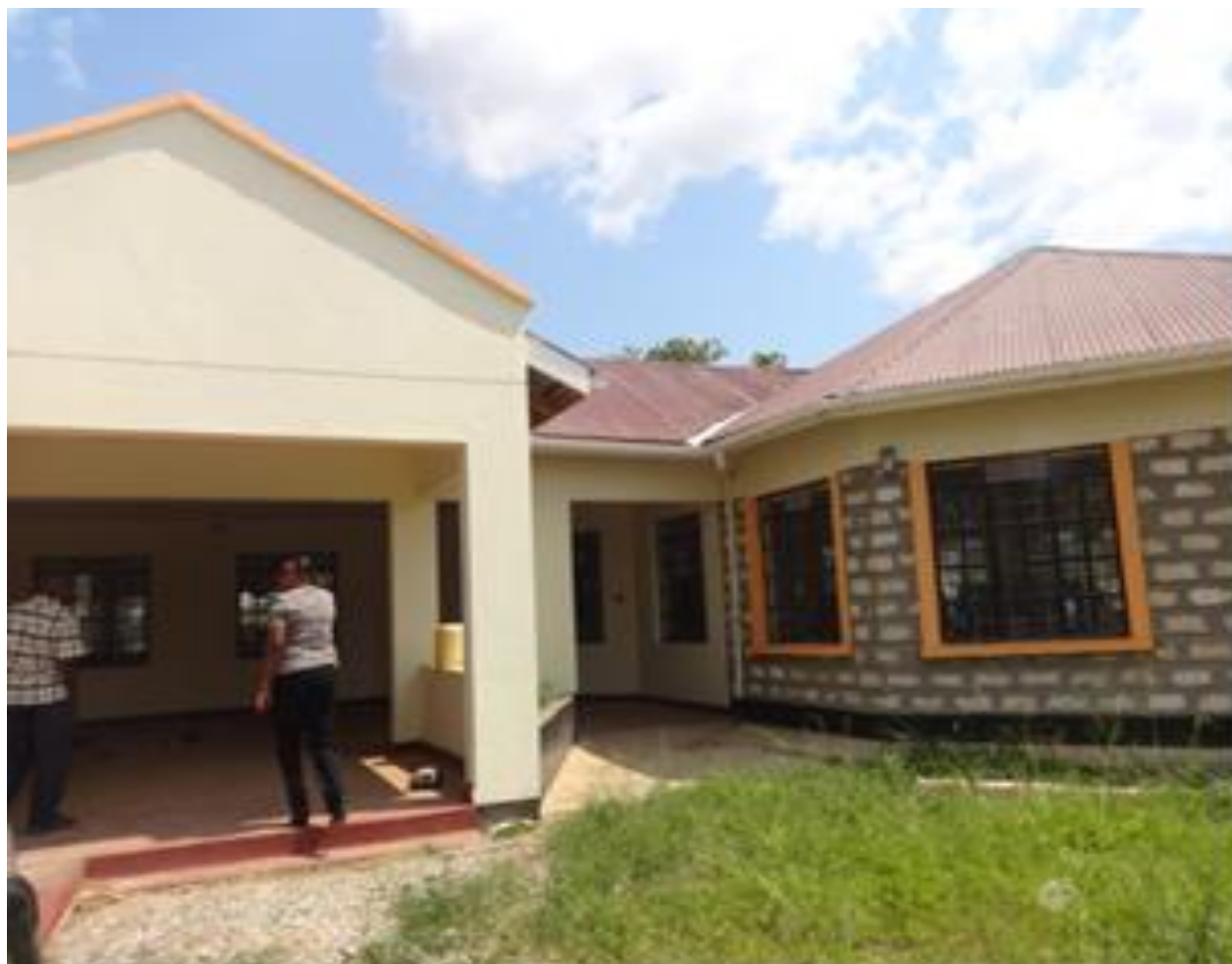
Public library in Kinango constructed and equipped by the County Government
