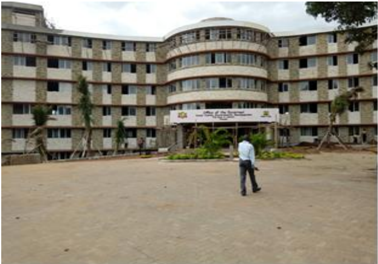
The newly constructed county headquarters in Kwale town
