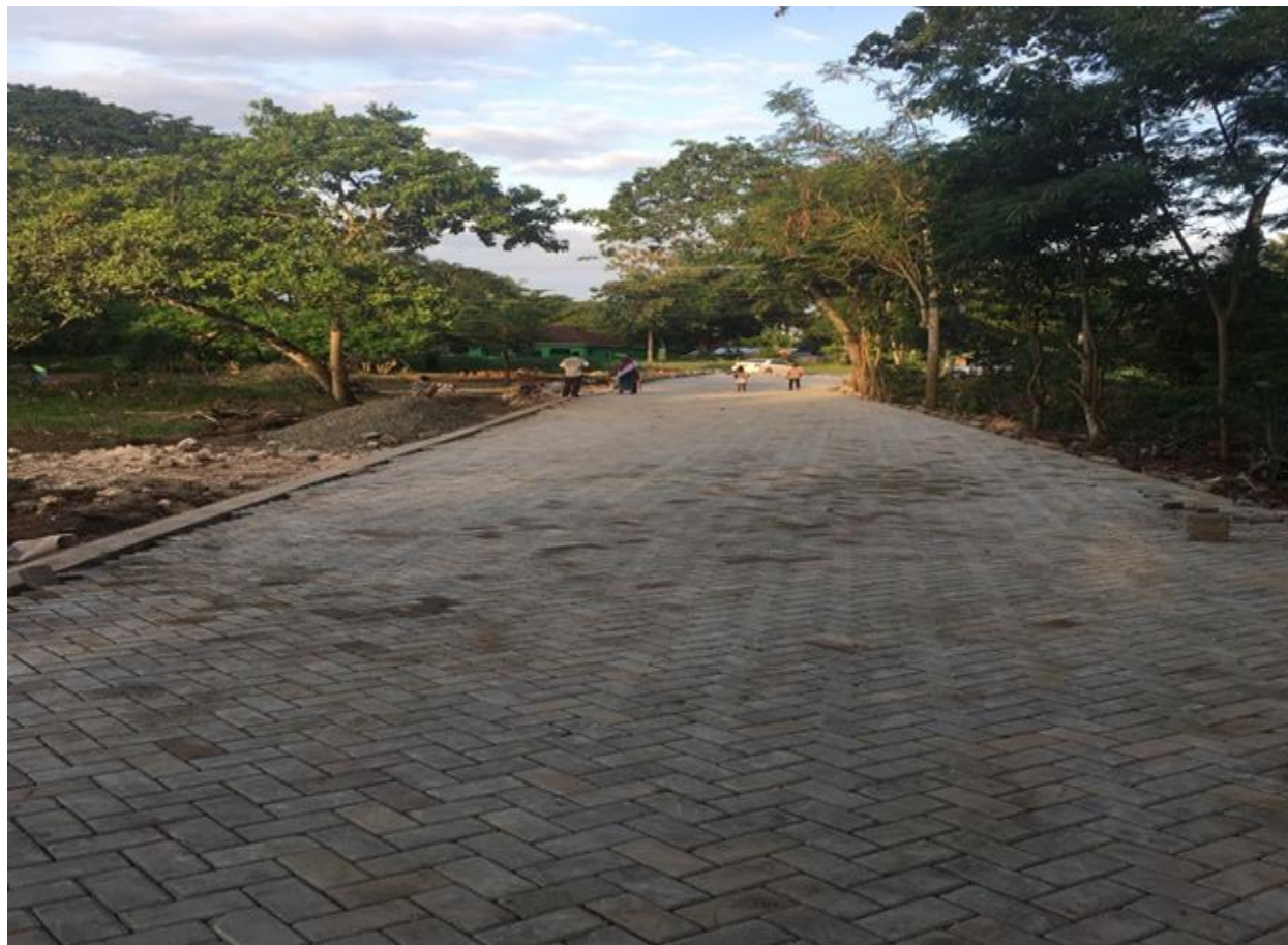
Cabro laying of the Pungu Slaughter house access road
