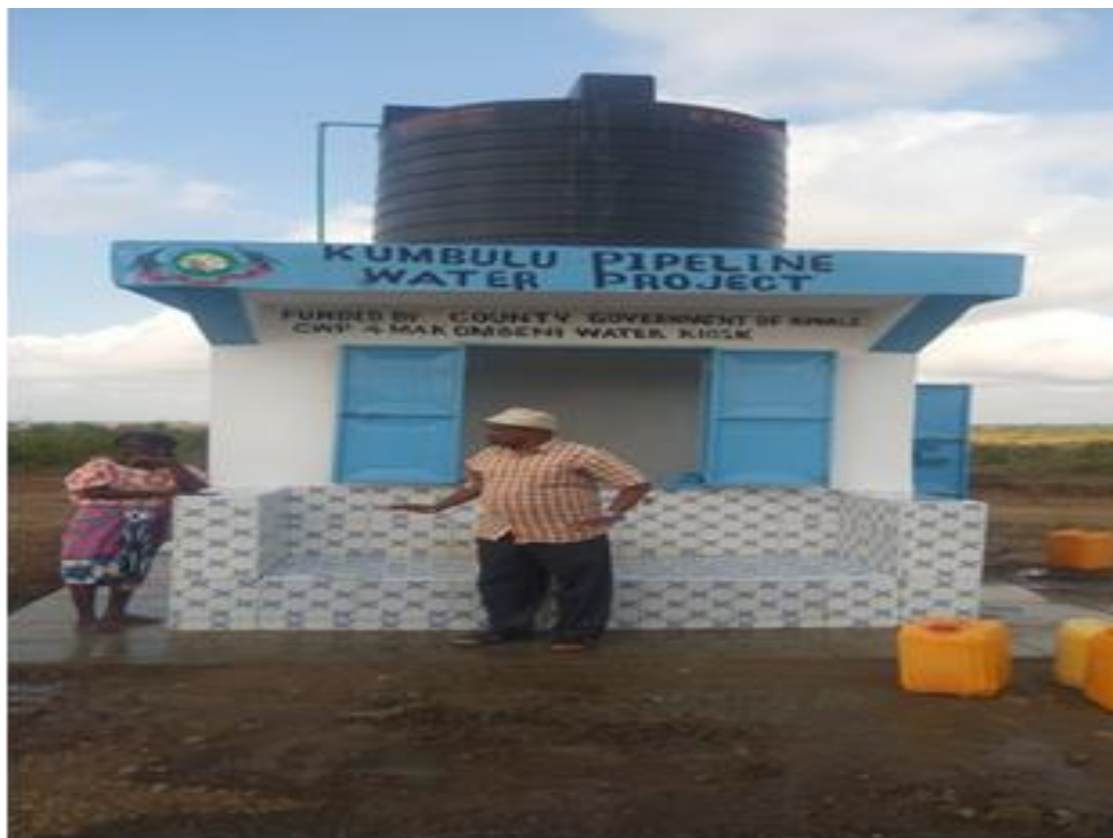
Kumbulu water pipeline project in Makongeni- Waa-Ng'ombeni ward
