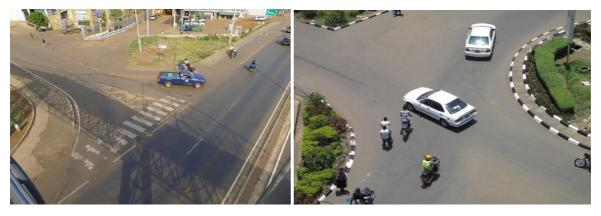
Figure 18: Wide turning radii at intersections encourage speeding by vehicles, thus making it unsafe for pedestrians to cross the road.
