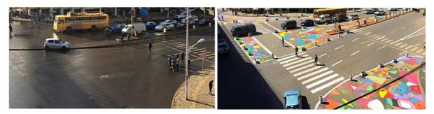
Figure 68. Before and after images of intersection modifications in Addis Ababa to reduce lane widths and turning radii for motor vehicles in order to improve pedestrian safety.
