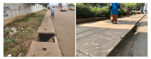
Figure 86: Loose drain covers make for a poor walking surface (left). A well-finished footpath on top of a major stormwater drain provides a comfortable walking surface (right).
