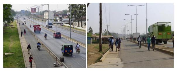
Figure 15: Wide shared lanes for pedestrians and cyclists along Nairobi-Busia highway. The NMT facilities are often encroached by motor vehicles, introducing safety risks for pedestrians.
