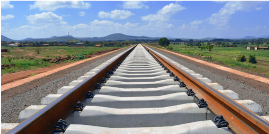
Figure 14: A Section of the Standard Gauge Railway
