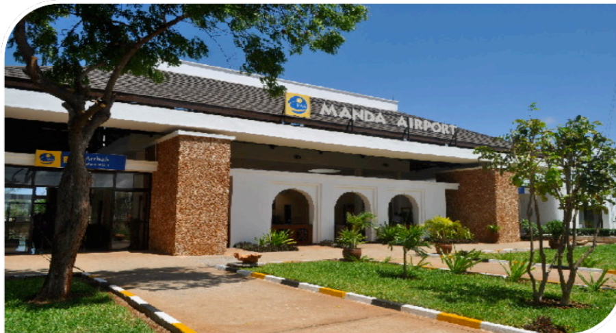
Figure 29: A Terminal Building at Manda Airport, Lamu County
