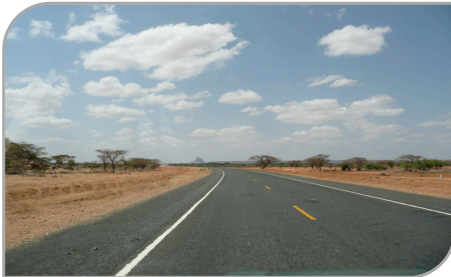
Figure 27: Part of the Completed 530km Isiolo- Moyale Highway
