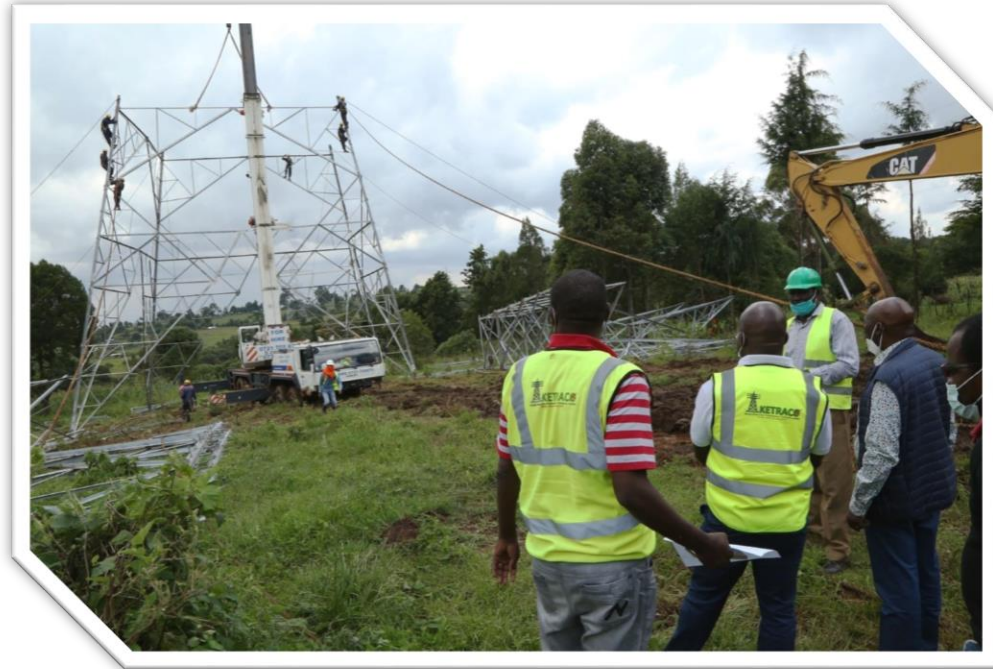
Figure 10: Construction of Olkaria-Lessos-Kisumu transmission line Source: KETRACO
