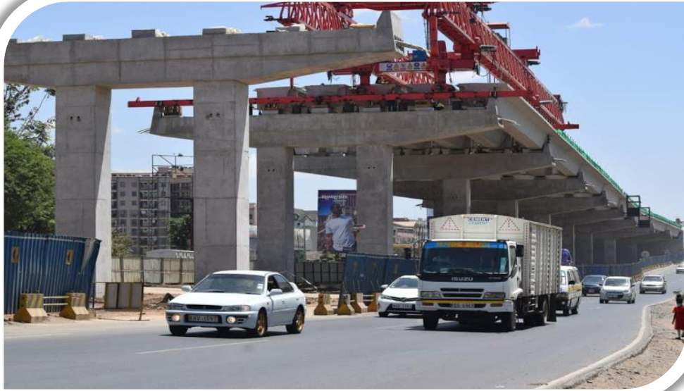
Figure 7: A section of Nairobi Expressway under construction Source: Kenya News Agency
