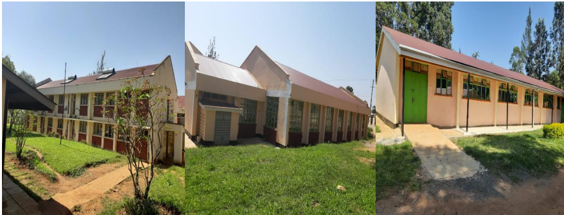
Plate 8: Refurbishment of mabanga ATC
