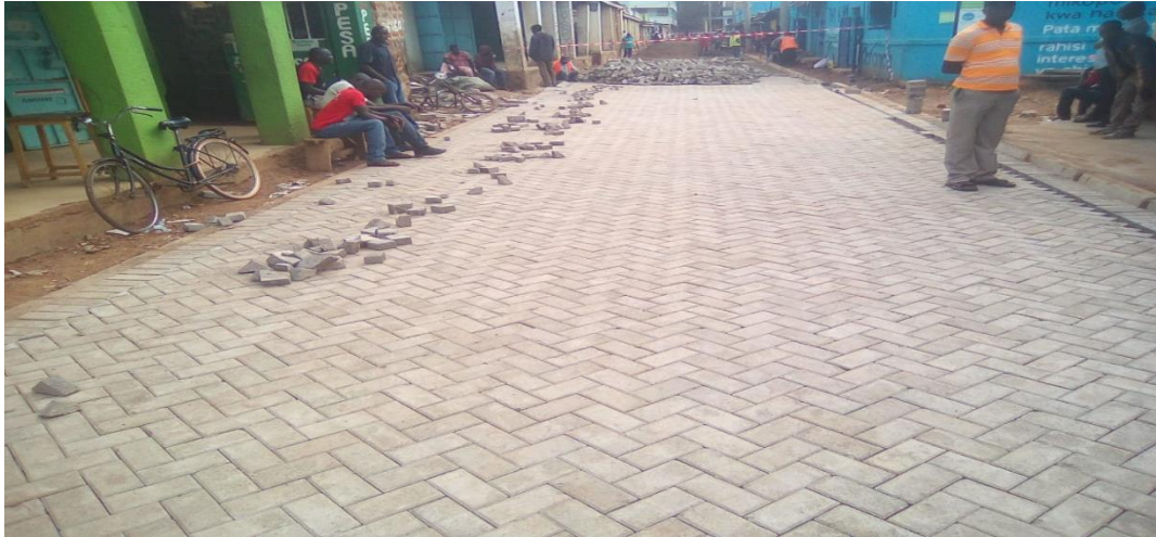
Plate 4: Upgrading a road behind cooperative bank road in bungoma town.
