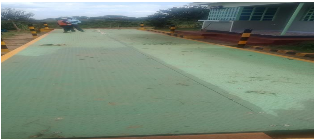
Plate 10: Digital Weigh Bridge at Musese coffee milling plant-
