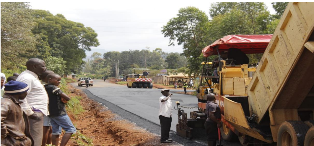
Plate 3: Upgrading Of Riziki-Dc ,Riziki To Slaughter House Road In Kimilili Municipality.
