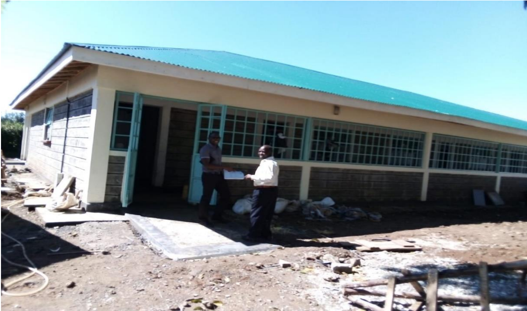
Plate 1: Bumula sub county theatre under construction
