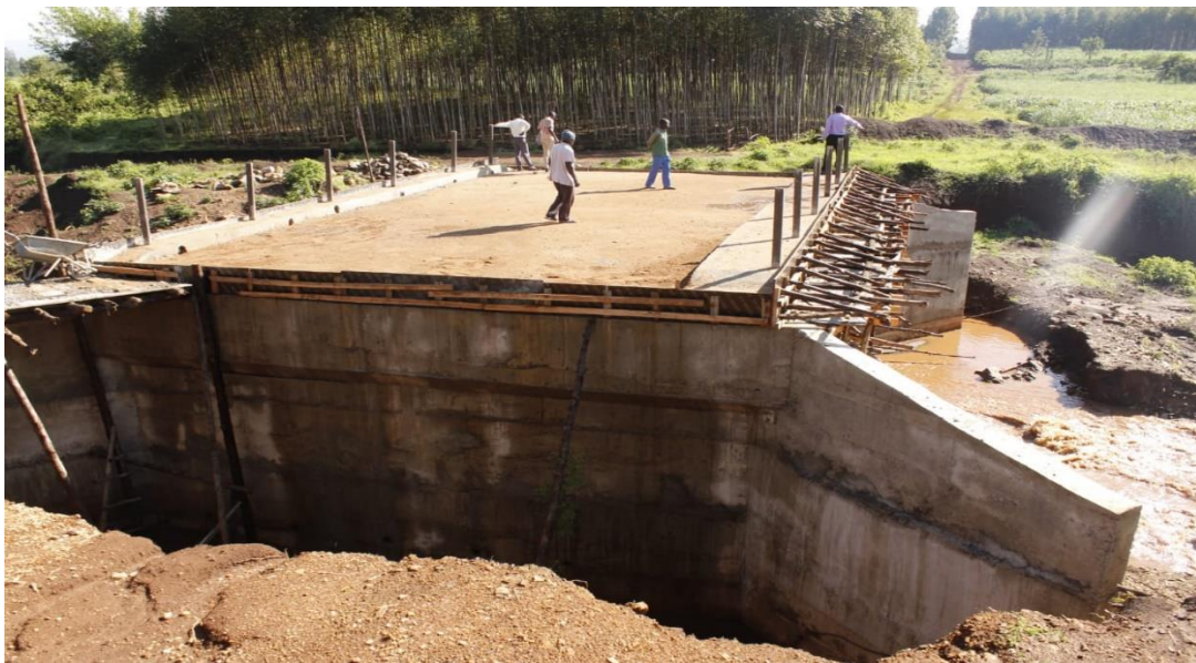
Plate 5: Bridge building at Mausobunang,ani Bokoli in Webuye west Sub County.
