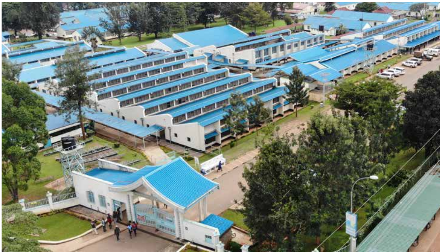
Photo 7: The Kakamega County General Hospital (CGH) in Lurambi Sub-County
