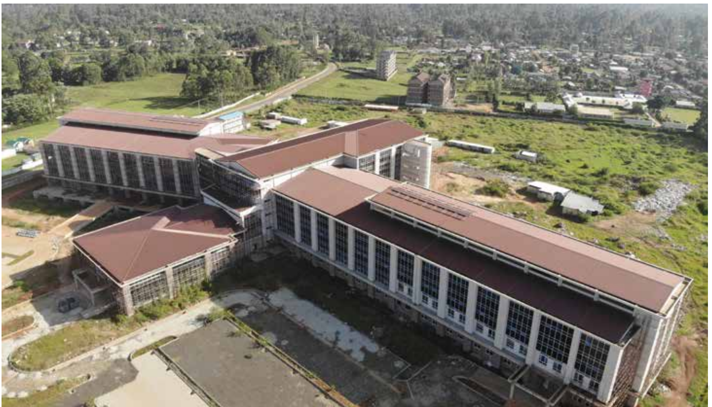
Photo 21: Ongoing construction of Kakamega County Teaching and Referral Hospital (KCTRH)
