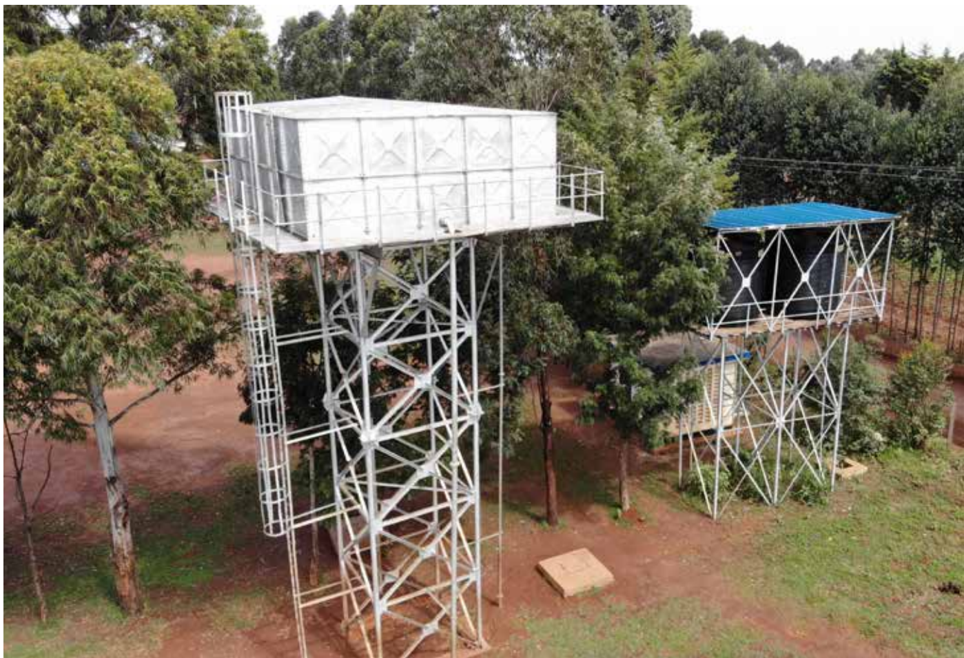
Photo 9: A 50,000m 3 elevated steel water tank at St. Monica community area in Likuyani Sub - County
