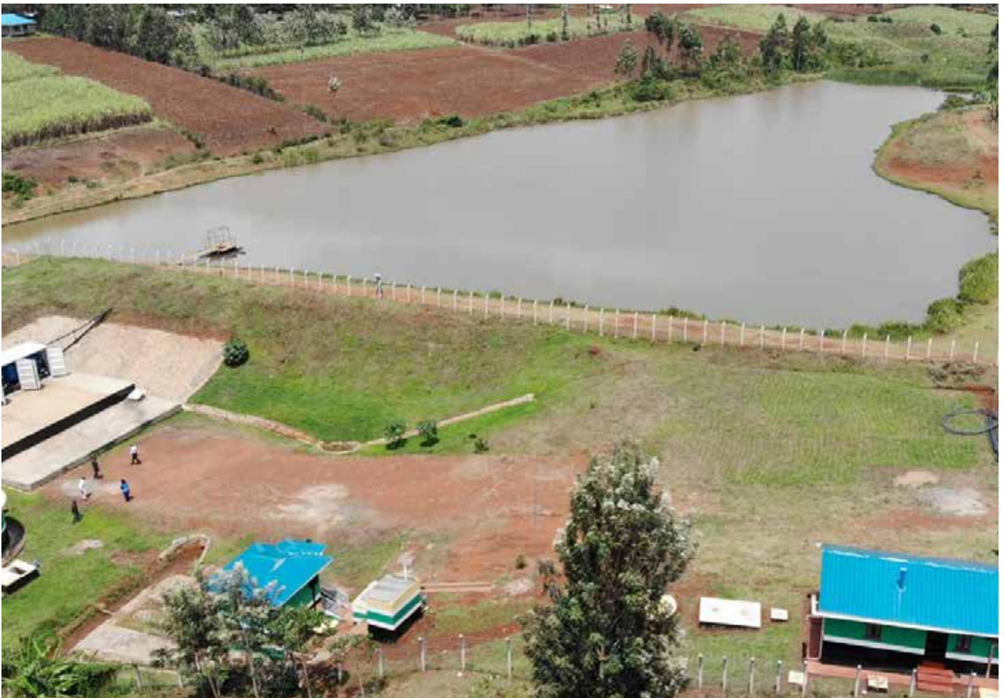
Photo 23: A 40 feet containerized water treatment plant with a production capacity of 100m 3 of portable water at Musembe dam in Chekalini Lugari Sub-County
