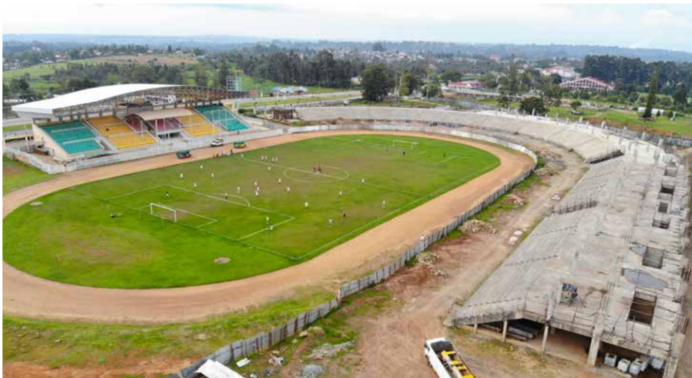
Photo 28: Ongoing construction of Bukhungu international stadium in Kakamega Town
