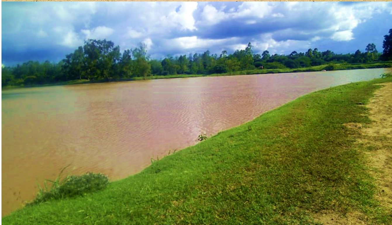
Photo: Miangeni Earth dam, Kivaa Ward
