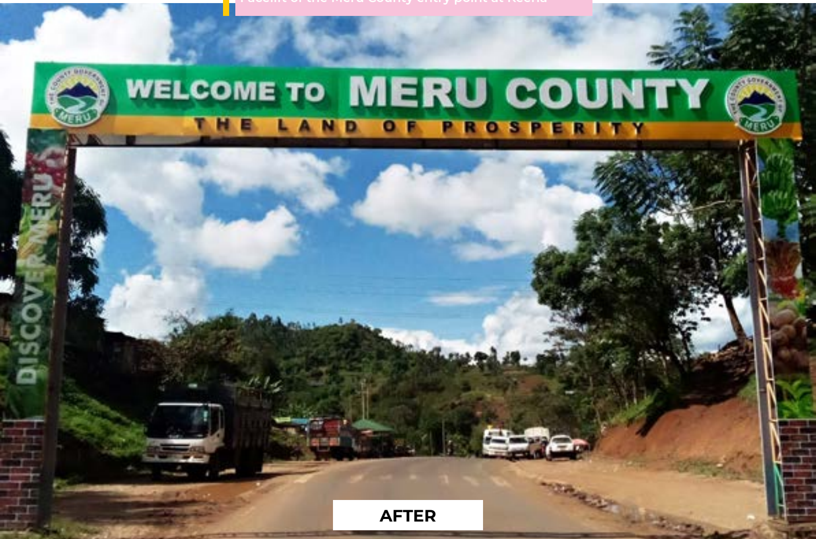
Photo No: 11 Facelift of the Meru County entry point at Keeria
