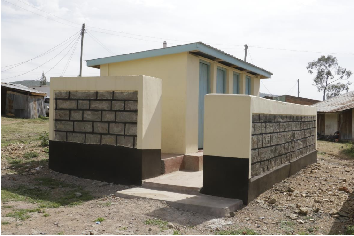
Plate 21: Okanowach Market toilet in West Nyakach Ward
