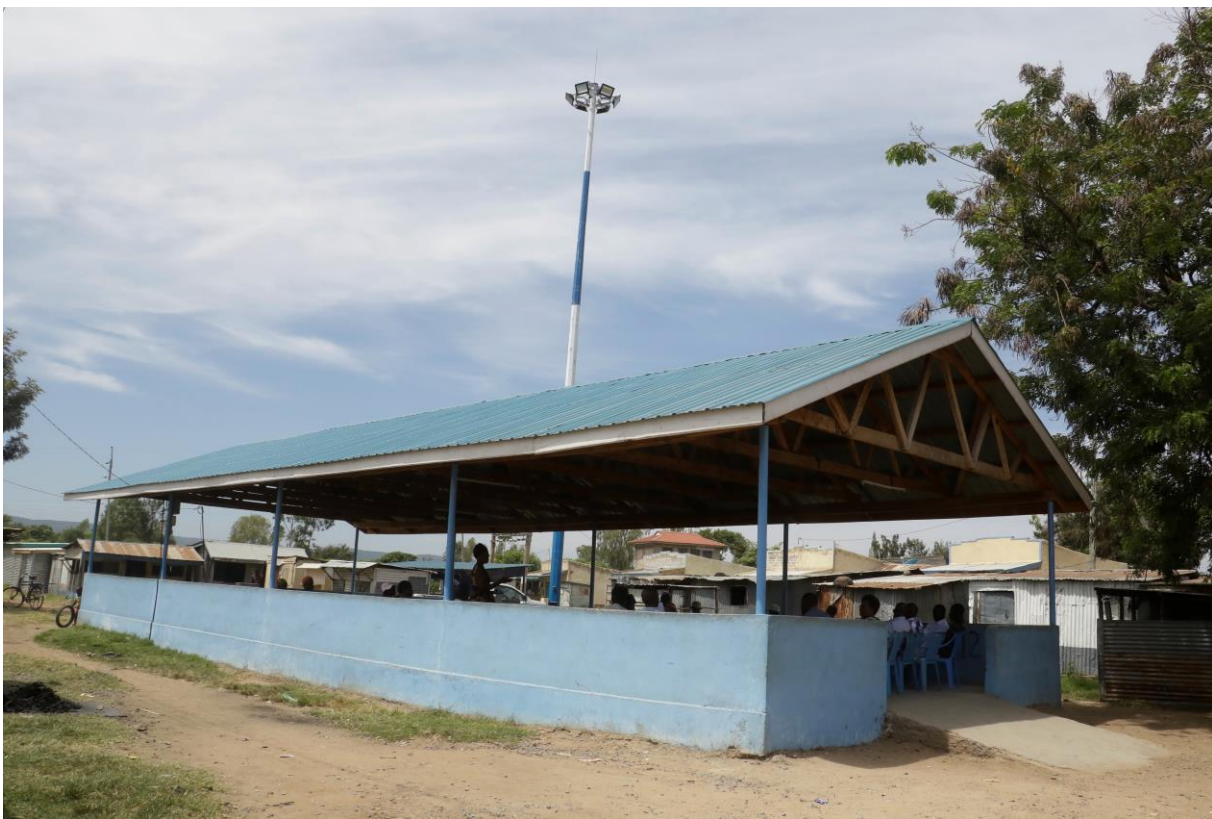
Plate 20: High mast flood light at Sango-Rota Market in West Nyakach
