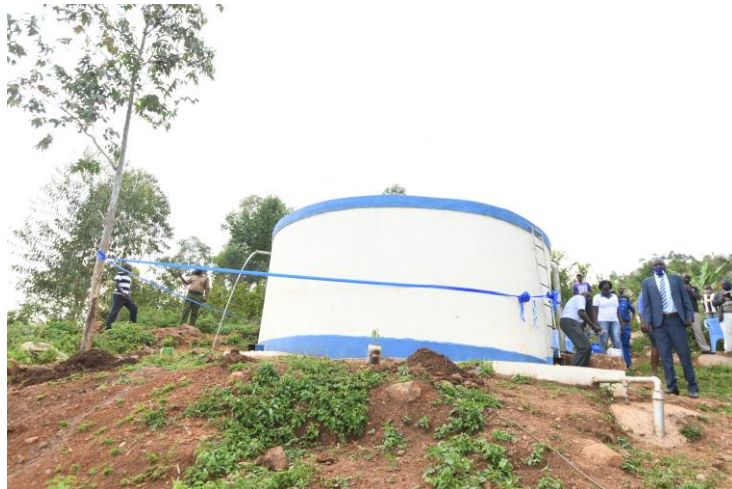
Plate 18: Esivalu Water Project in Maseno, Kisumu West Sub-County
