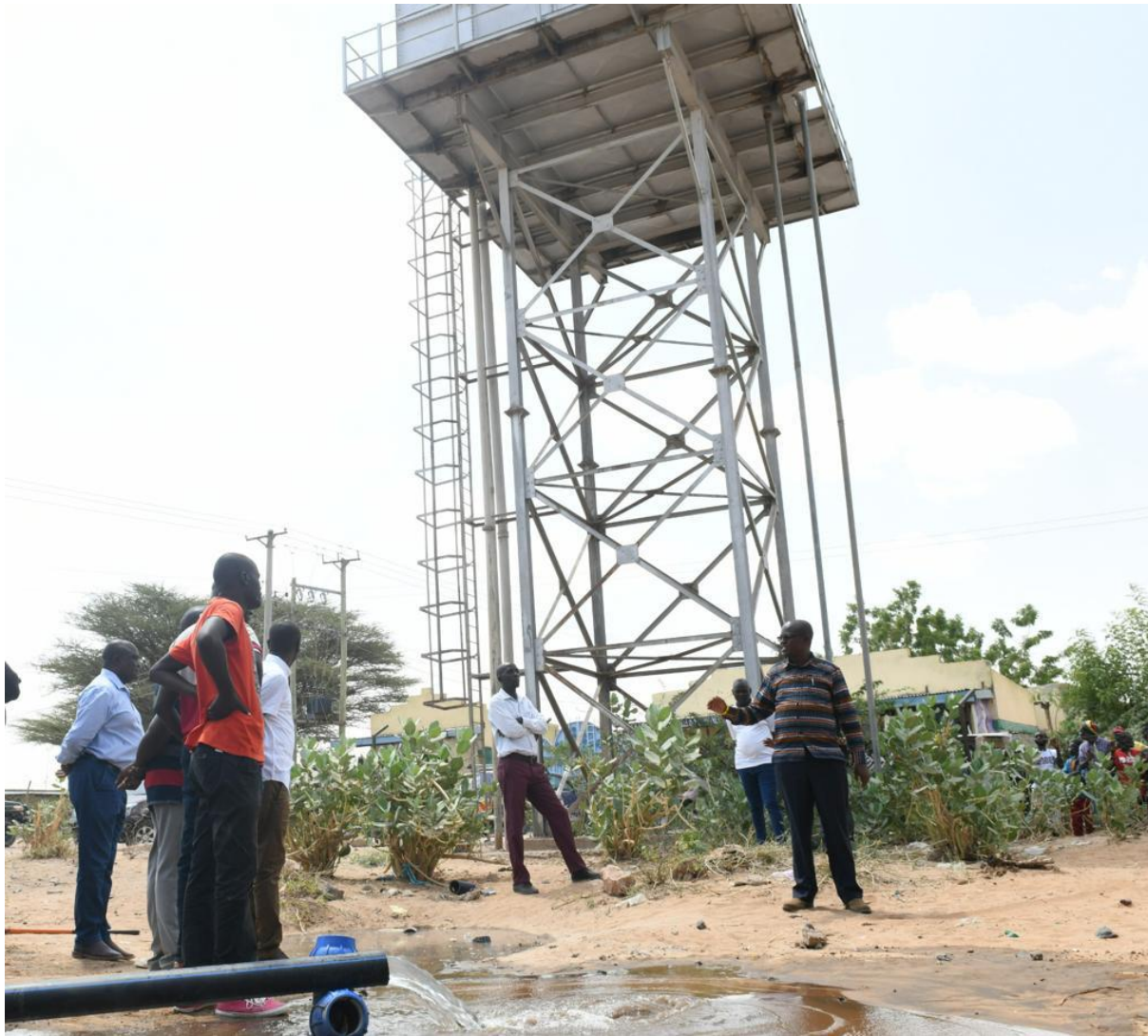
County Water Project in Kanamkemer ward.
