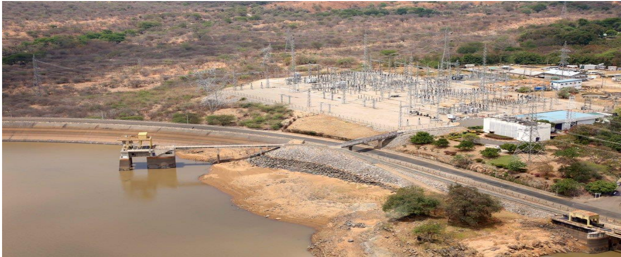
Figure 5b: Masinga Dam
