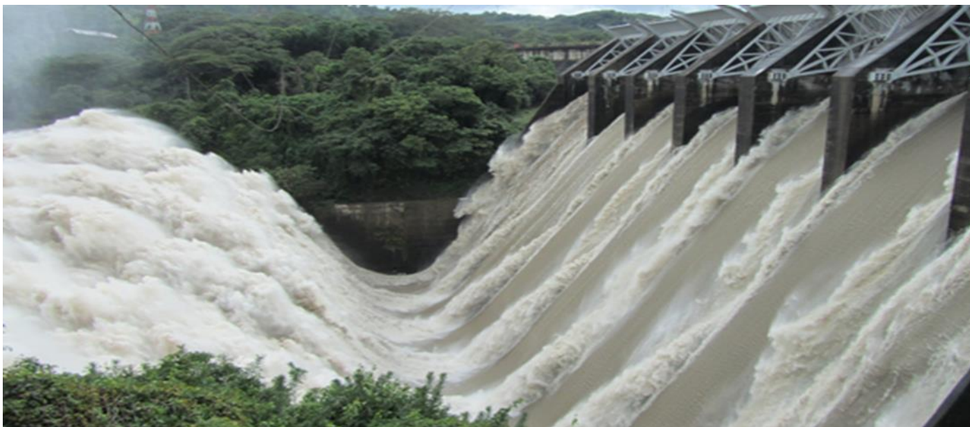
Figure 5a: Hydro Electric Power Dams
