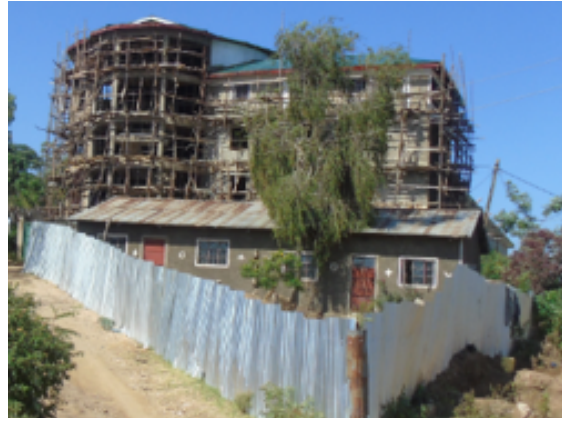
Modern apartments under construction in Kibabii
