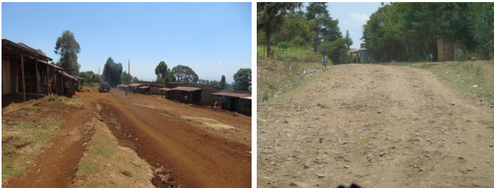
Picture 4: Poor road conditions in Naitiri and Nabuyole
