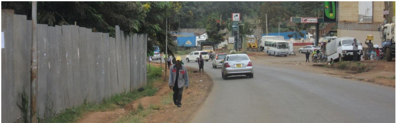
Figure 57: Poor road condition in the wet season
