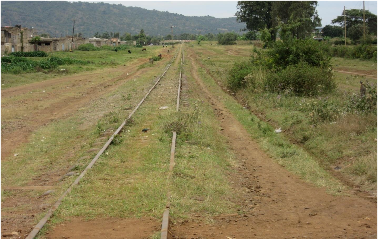
Figure 54: Abandoned railway line near Muragua
