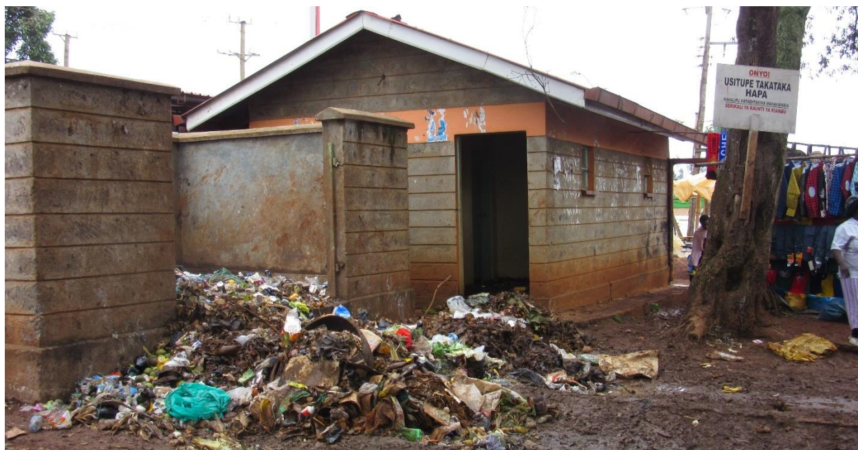
Figure 66: A lack of ablution facilities and waste removal at markets
