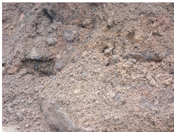
Unconsolidated soil leading to unstable slopes when disturbed (Outside Murang’a town)
