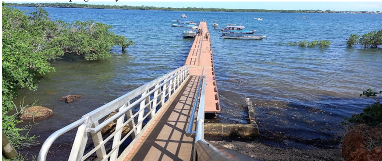
Kisite Mpunguti Jetty links Shimoni to Wasini Island in Kwale County
