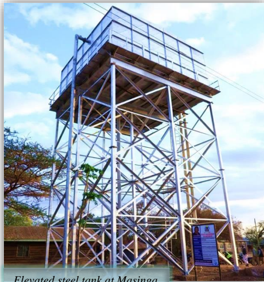
Elevated steel tank at Masinga
