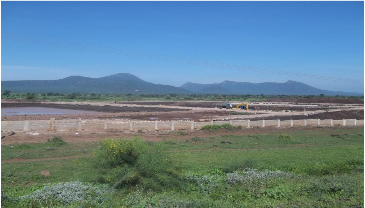
Figure 11: Expansion Project of Sewerage Ponds in Isiolo Town
