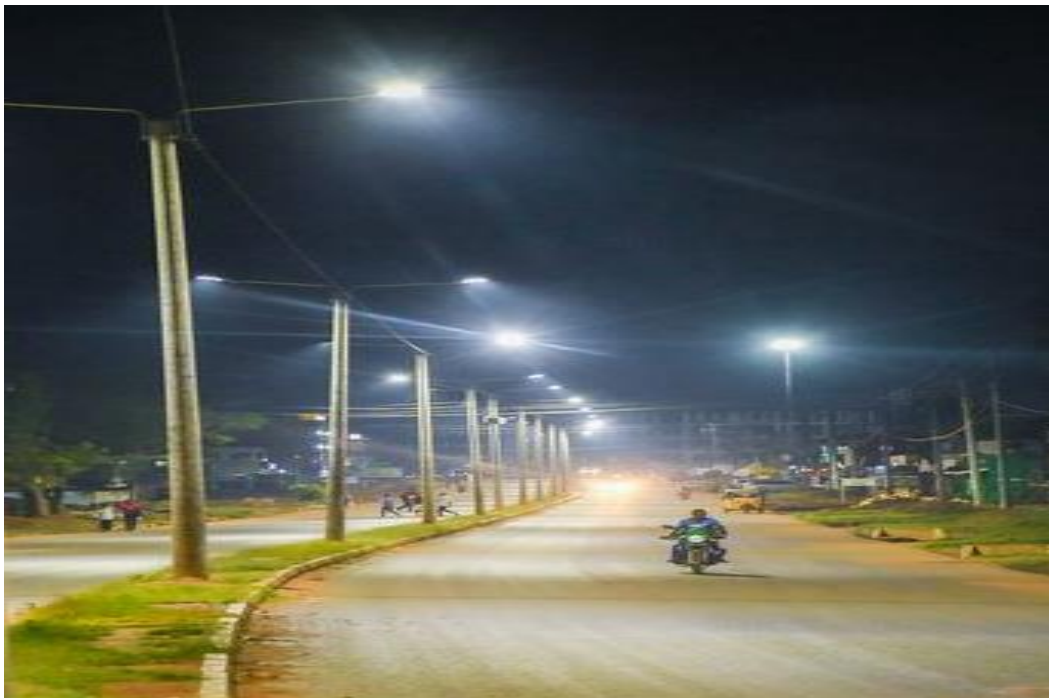
Figure 10: Sangalo Junction – Kanduyi Dual Carriageway (6.5km)
