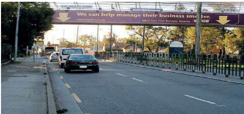
Does not detract from architectural elements of bridge; does not block views; advertising form compatible with bridge form.
