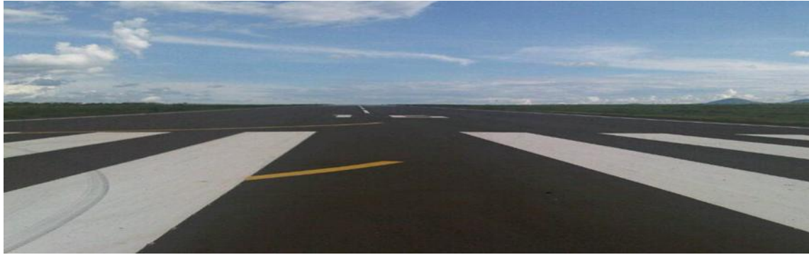
Figure 5: Completed 1.4km Runway in the first Phase of Isiolo International Airport, 2018
