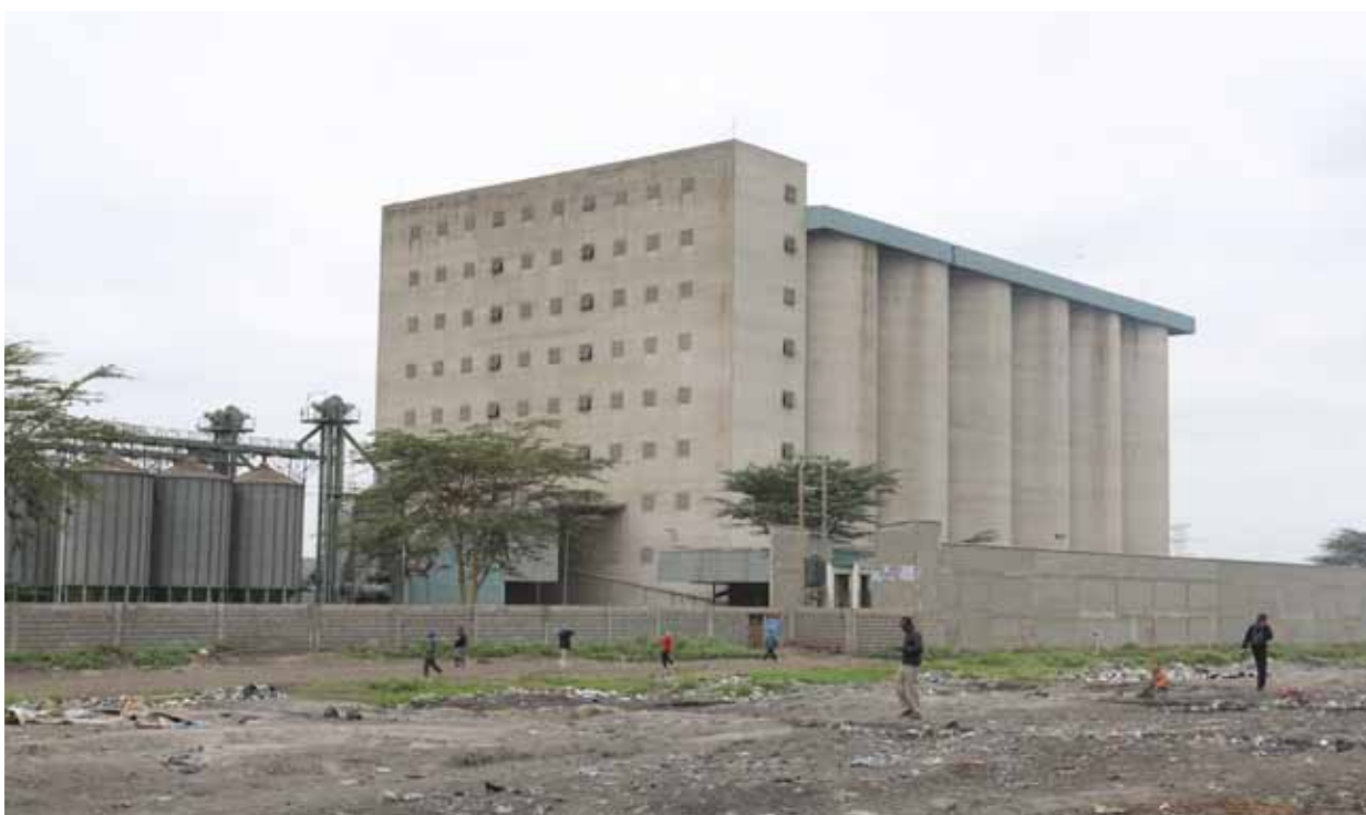
National Produce and Cereals Board grain storage facilities on Outer Ring Road, Nairobi
