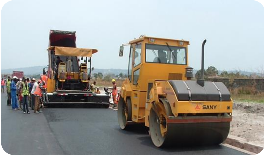
Figure 6: Road Maintenance Project in Progress
