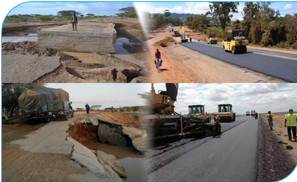
Figure 21: Rehabilitation of key infrastructure
