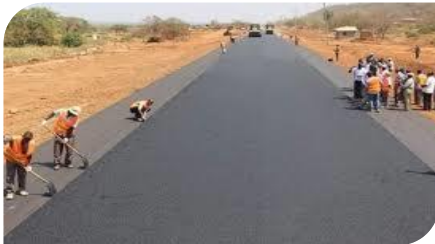
Figure 22: Construction of the Kibwezi- Mutomo- Kitui Highway
