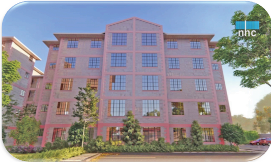
Figure 3: 250 Housing units in Kanyakwar, Kisumu County Source: MDA Reports, 2018
