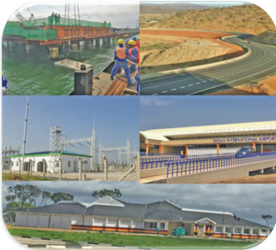
Figure 21: Ongoing Lapsset Project
