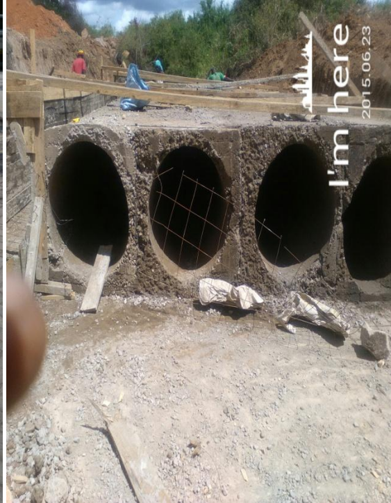
Chakama Drift Construction Works
