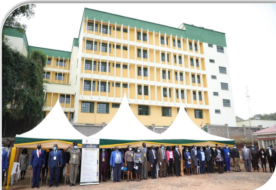
Figure 7: Hon. Chief Justice and staff during the opening of Kapenguria Law Courts Complex Source: Judiciary Report, 2021
