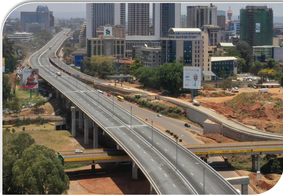
Figure 12: A section of the Nairobi Expressway under construction Source: KeNHA, 2021
