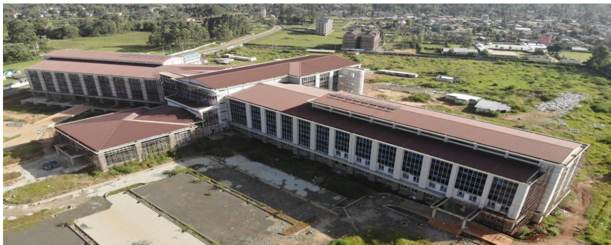
Photo 1: The new Teaching and Referral Hospital under construction in Lurambi Sub-County
