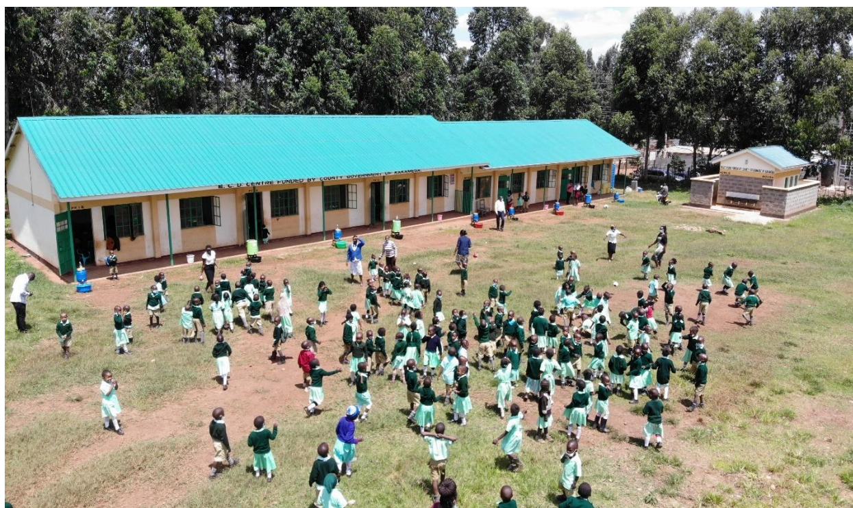
Photo 2: Kakamega primary ECDE Centre. The County government has constructed 316 ECDE Centres across the County
