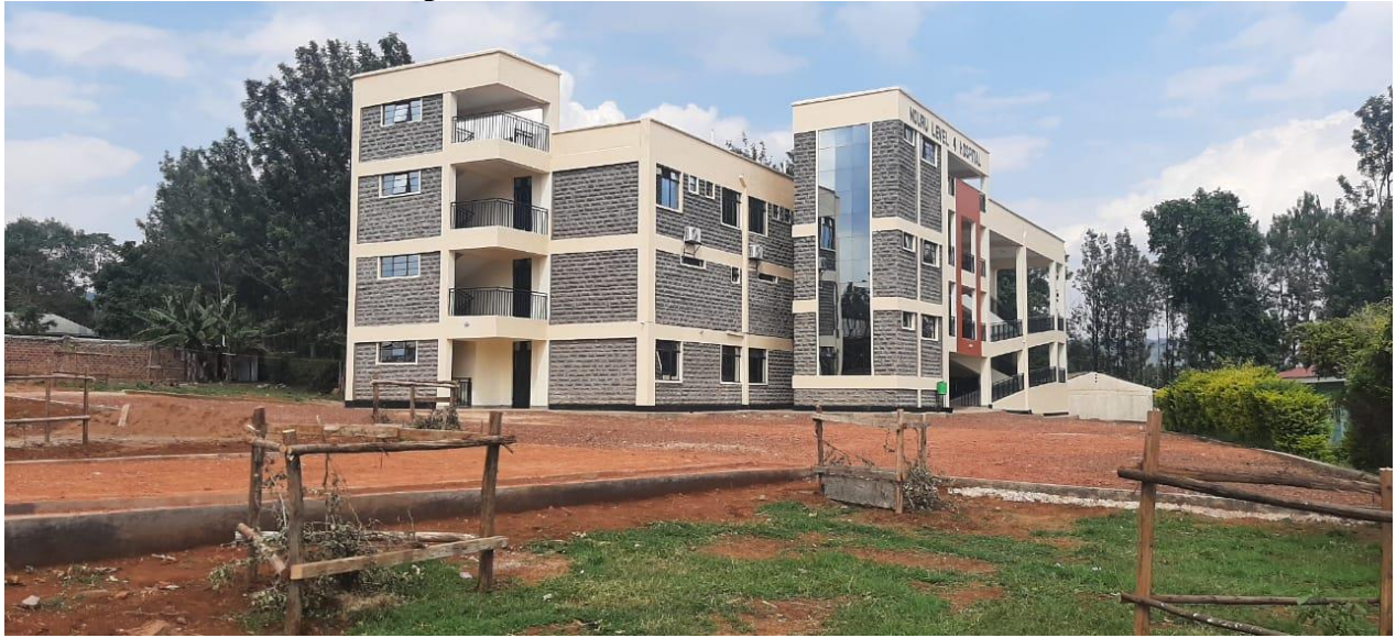
Photo 5: Nduru Level 4 Hospital
