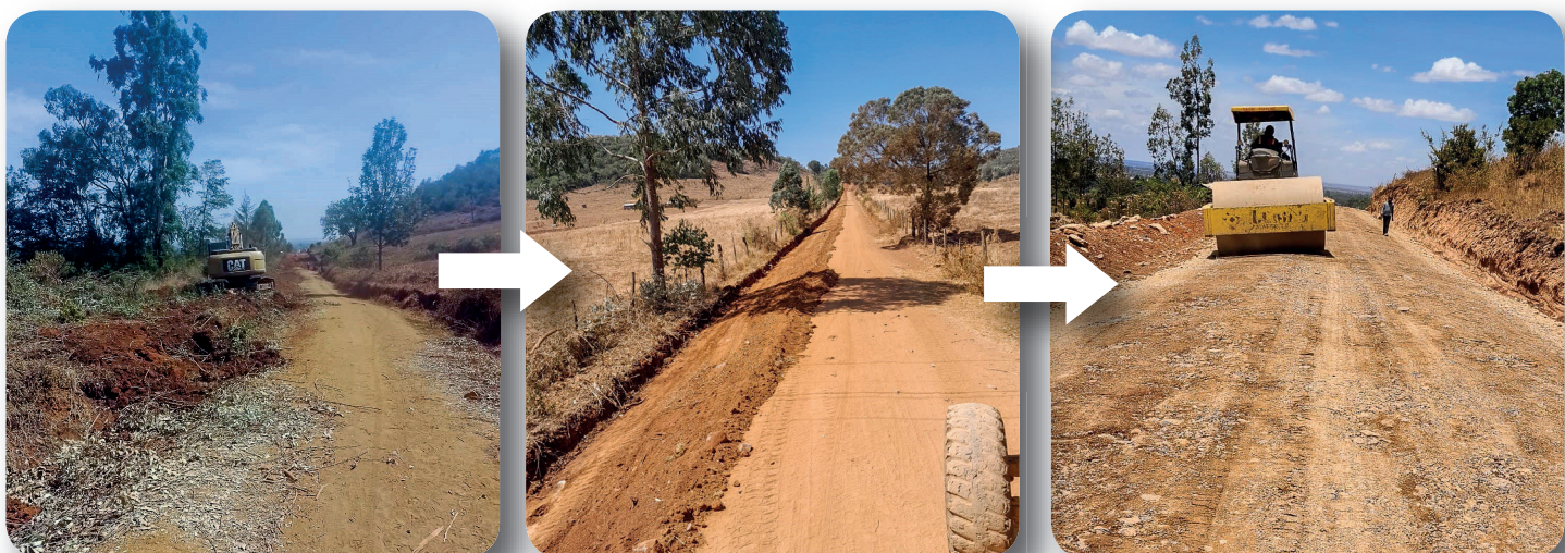
Grading and graveling of the Ndurumo - Karage Road
