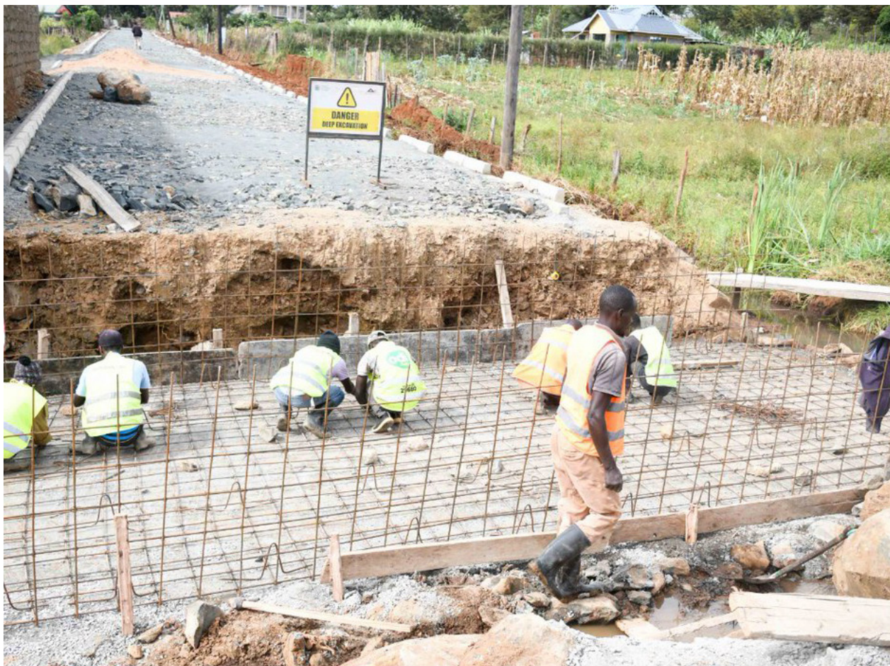
Installation of culverts in residential areas in Laikipia County
