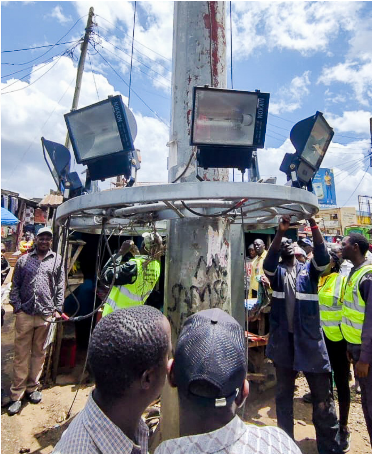
Installation of high-mast floodlights in urban areas in Laikipia County
