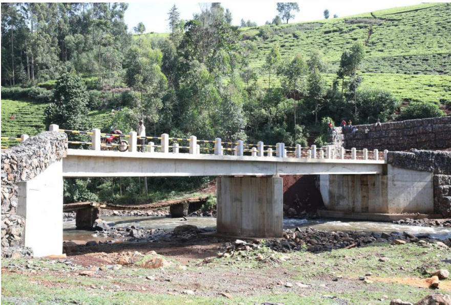
Plate 4: Construction of Muriaisai Bridge in Konoin Sub County
