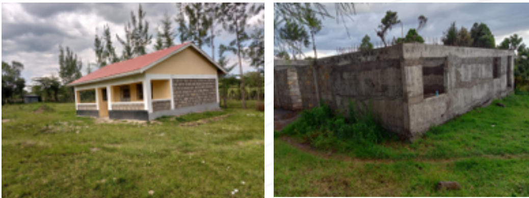
Plate 6: Kamundugi Dispensary and X-Ray Unit under construction in Tegat
