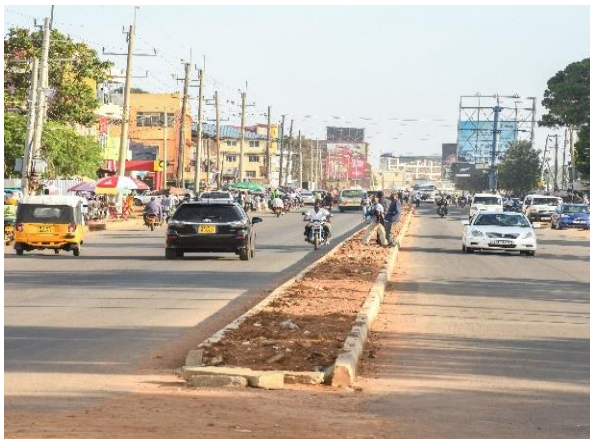
Dual carriageway road in Bungoma Town
