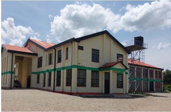
Dairy Processing Plant Structures at Webuye
