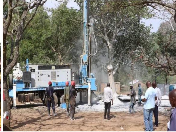
Drilling of Siloba Water Borehole in Kimaeti Ward
