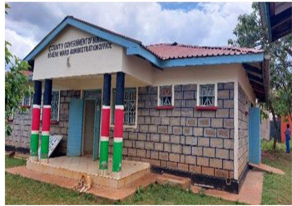
Maeni Ward Administration Office
