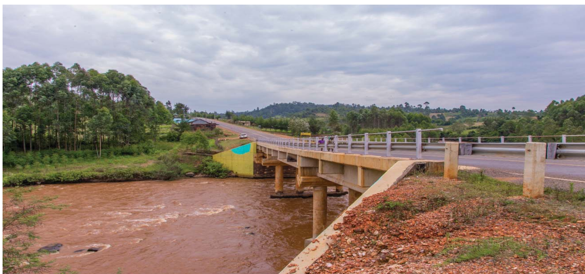
Figure 15: Bridge easing circulation due to connectivity
