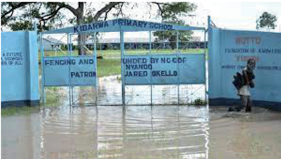
(c) Flooded Kibarwa Primary School in Nyando Plains (Photo/PD/Viola Kosome)
