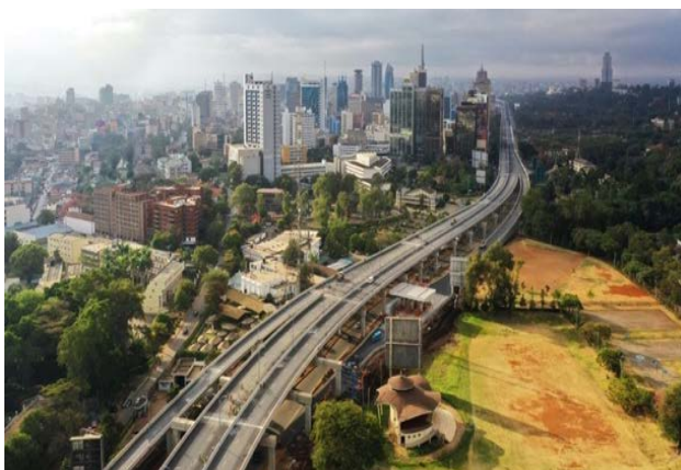
(b) The Nairobi Expressway
