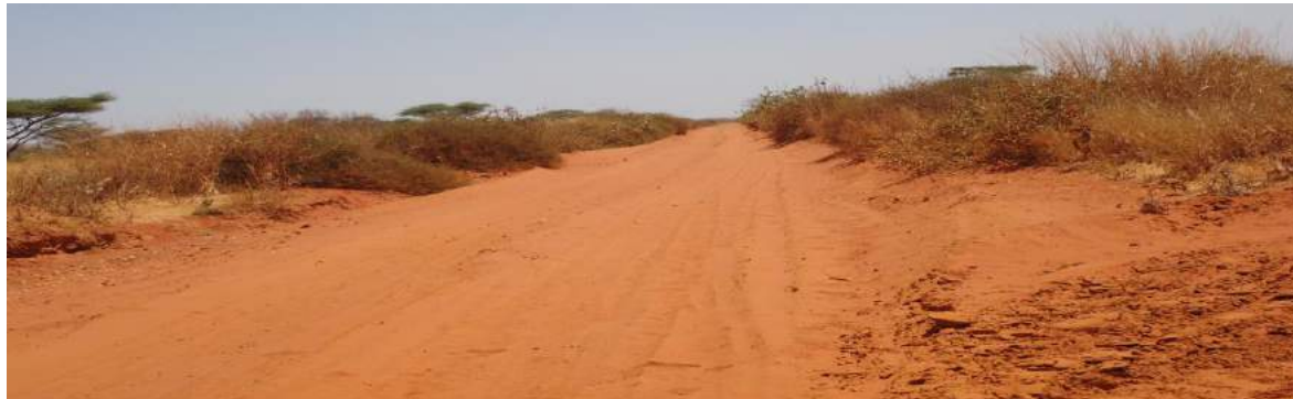
Figure 5: Earth road section along Mandera Town – Lafey Road
