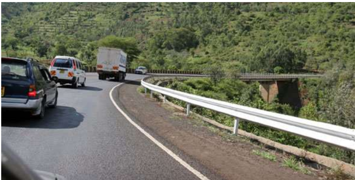
Picture 1: Nithi Bridge
