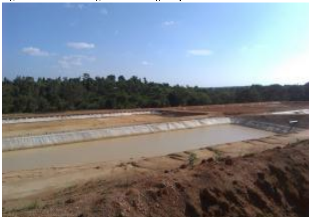
Figure 13: Kitui Sewerage Plant nearing completion
