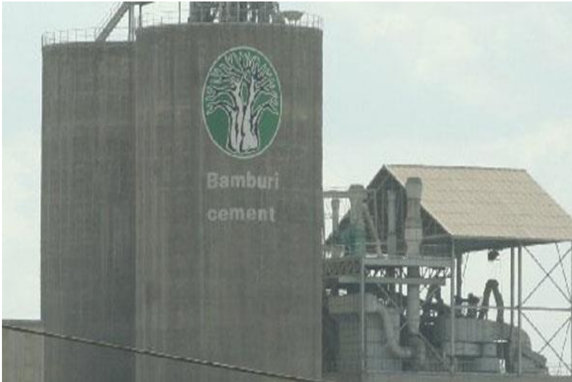
Bamburi Cement factory in Athi River
