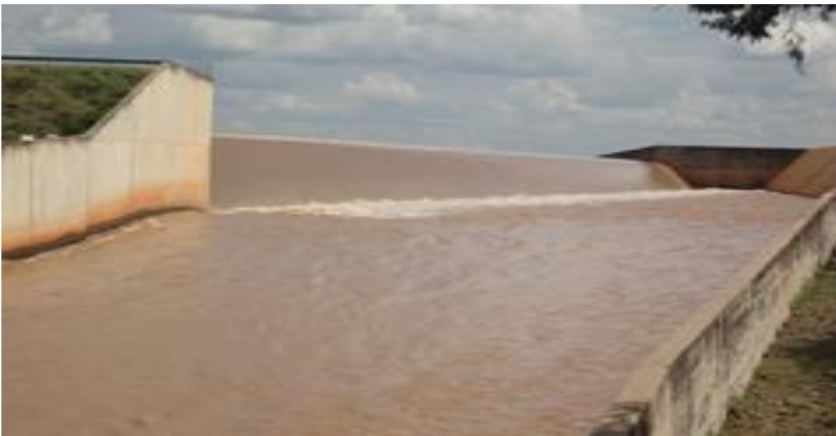
Masinga Dam Hydro-electricity power station.
