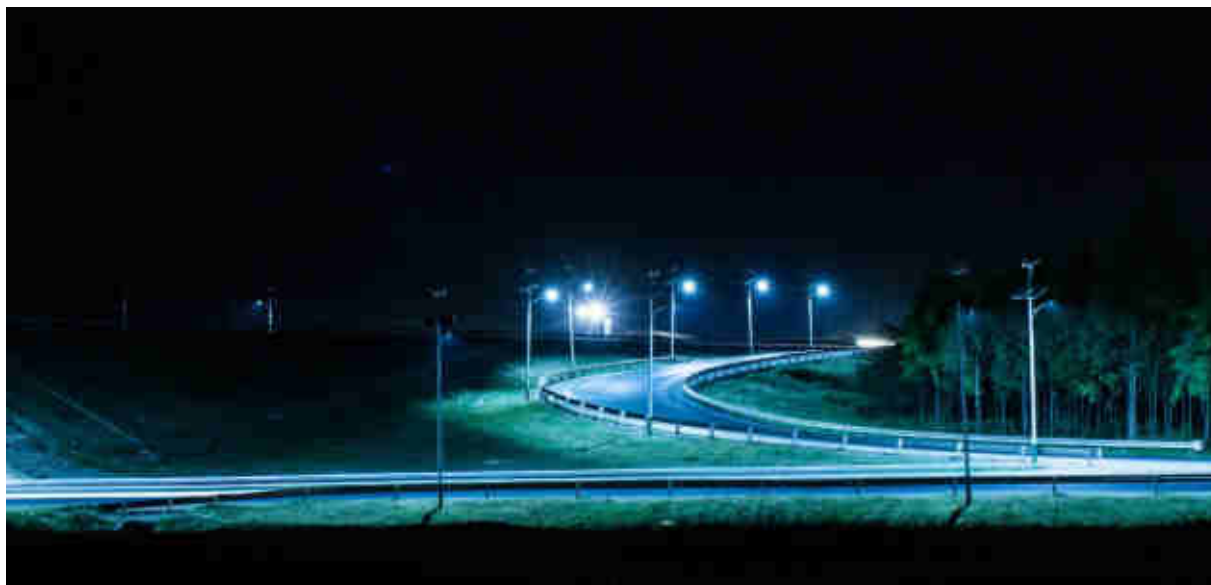
Namanga road interchange
