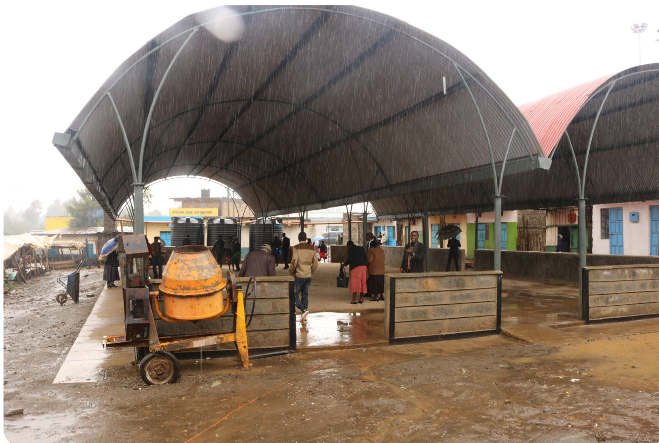
Ongoing construction of Njabini Market.
