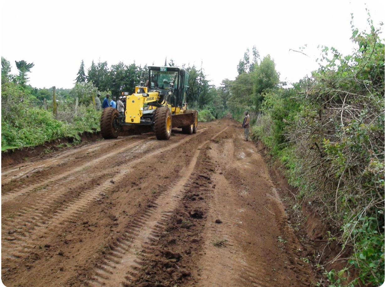
Ongoing gravelling of roads across the County.
